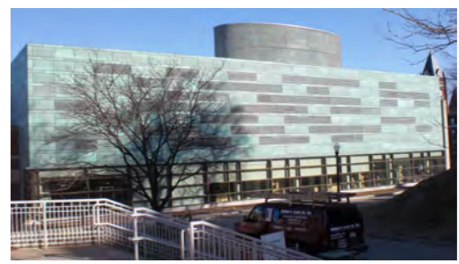
Copper panels at Holy Cross
