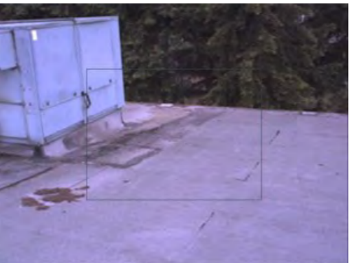
Camera image of roof area
