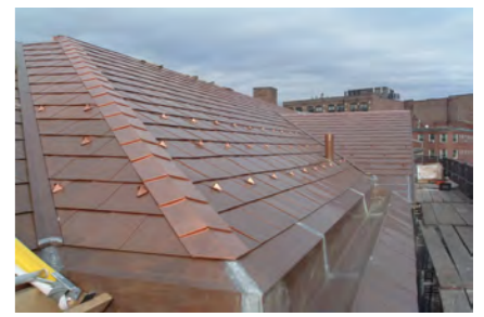
copper shingle roof at 128/152 north street
