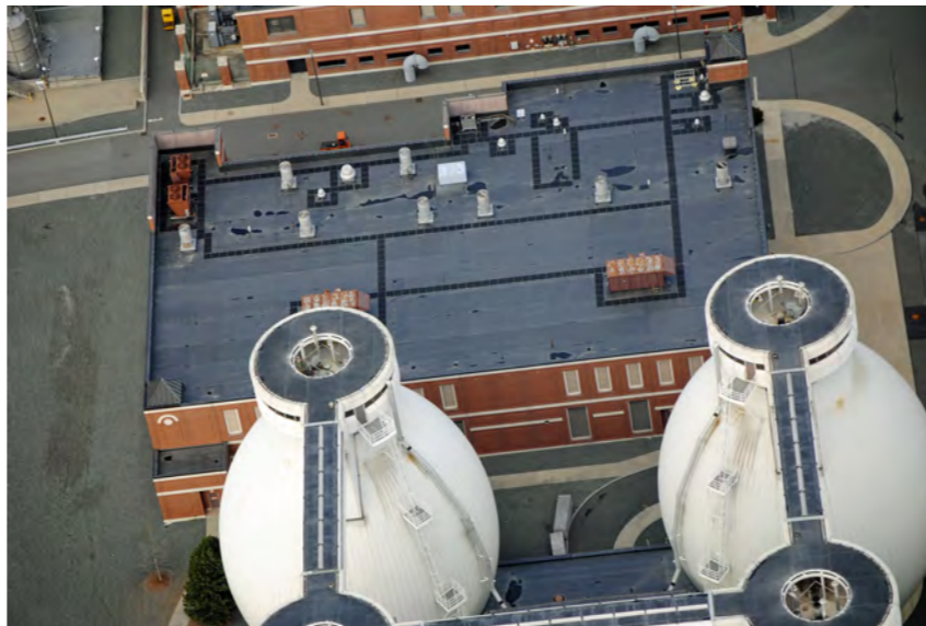
Deer Island treatment plant
