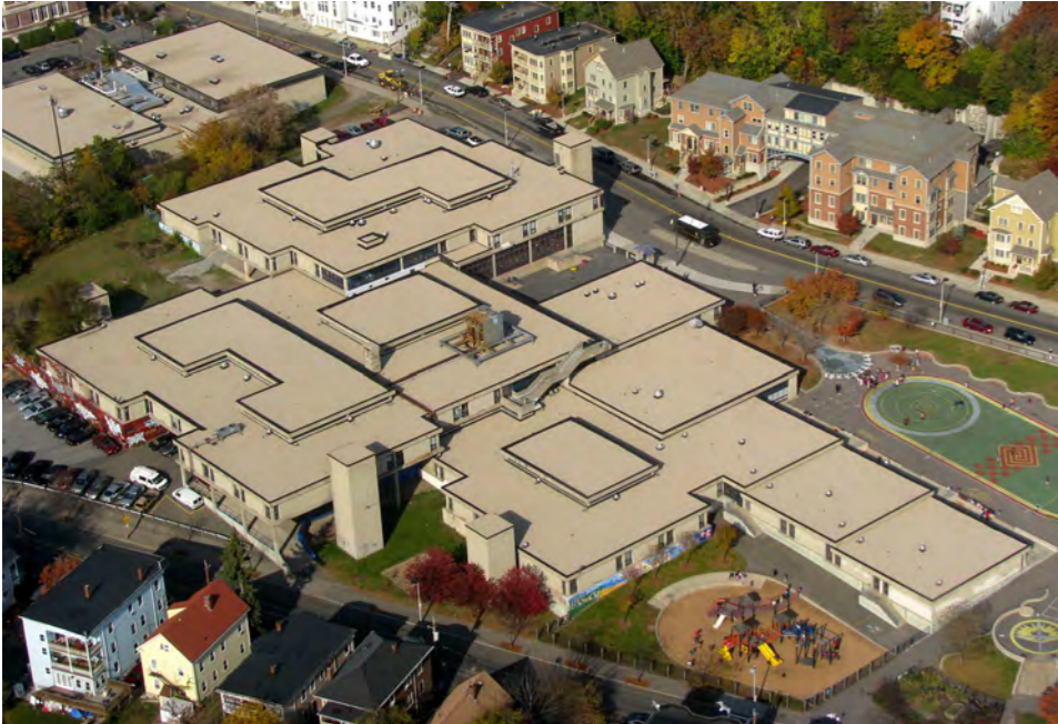
Hennigan Elementary School roof replacement.
